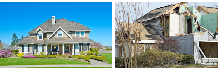
Two houses in need of renovation. The house on the left is in much better shape and as a result the renovation is much more likely to go smoothly and come in under budget.
